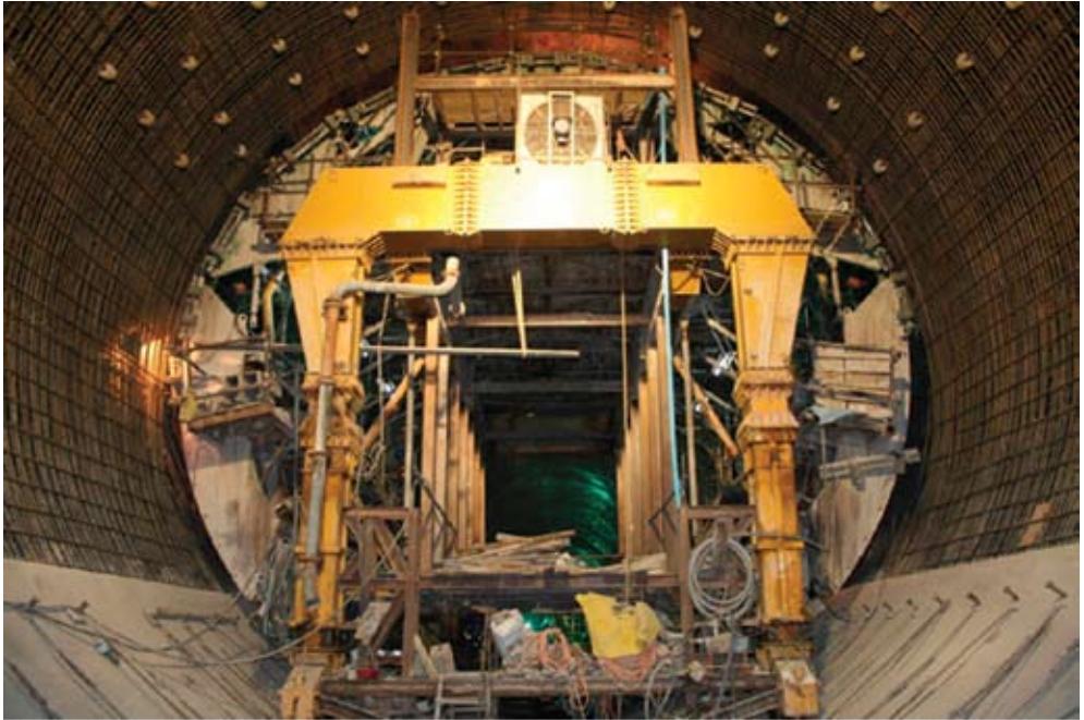
Picture 1. Shutter assembly for supporting a concrete lining to be poured inside of the tunnel
