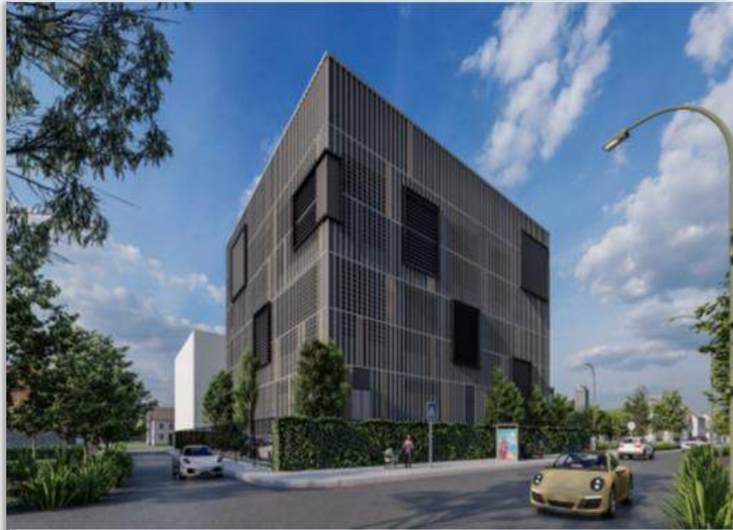
The Concession Contract for District Cooling Project for the Property Management of Chulalongkorn University Concession Period: 20 Years
