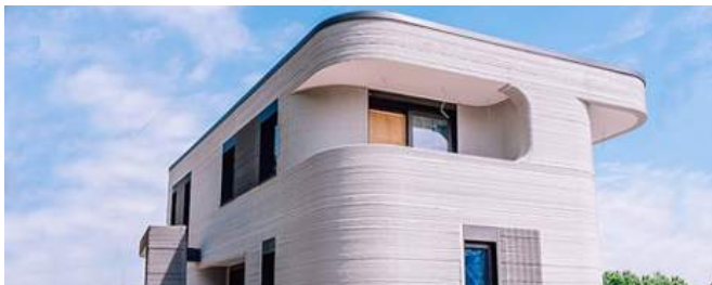
The first 3D-printed building in Germany, which took only 100 hours to complete. The building has a usable area of 380 square meters, and the only printed parts are the vertical walls. The floor and stairs are prefabricated at the factory. Ref: https://interestingengineering.com/germany-first-3d-printed-residential-building-is-near-completion
