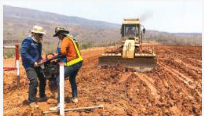
Inclinometer Installation
