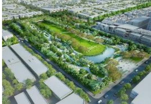
Water Recycling for the PMCU Contract Period: 10 Years Capacity 240 m 3 /day
