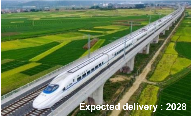
High-speed Rail Linking 3 Airports; EECO Project Management and Construction Supervision
