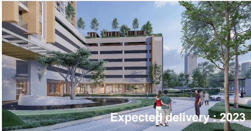
Detailed Design of the welfare building for the Secretariat of the House of Representatives
