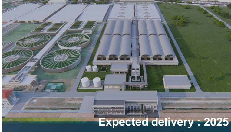
CSC of Mahasawat water treatment plant expansion to 800,000 cum/day and related work(Contract SV-901); MWA
