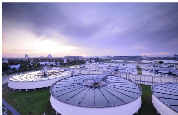
Water Supply Improvement Projects for MWA
