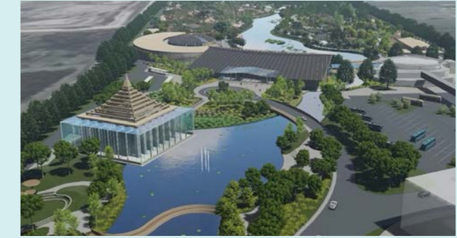
EPC work The New Zoo (Phase 1) at Khlong Hok
