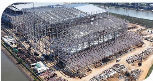
OMEGA Bangkna Warehouse Project: Pruksha Holding Public Company Limited
