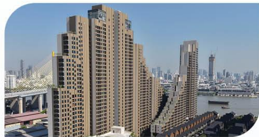
Skypark Lucean Jomtien Pattaya Project: Lunic Real Estate Company Limited
