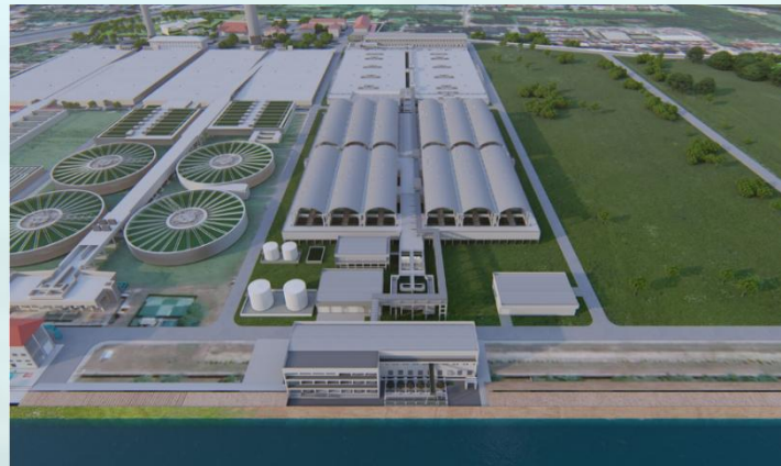
Drainage Tunnel/ Water Resources Management/ Water Supply/ Hydropower Projects
